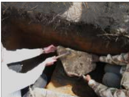
Jim tapping cornerstone into position
