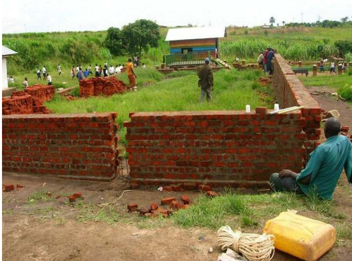
Construction of Mama Elsie's Chapel as of June 6.
